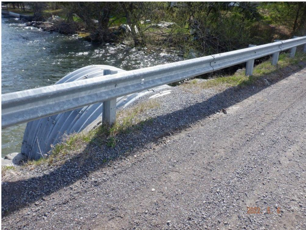
Railing system over culvert (typ)
